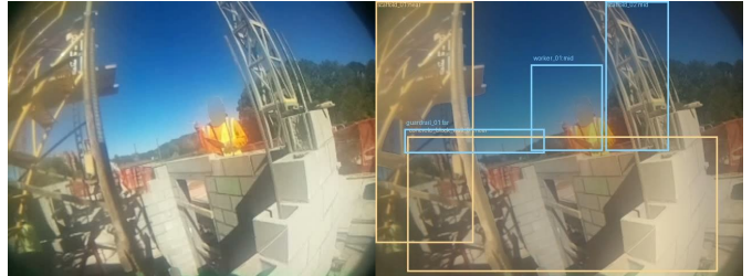
Figure 1: The basic VIMA evidence unit: a raw hardhat frame next to a depth-conditioned view. The depth map is not used as metric truth; it is used as an RGB-derived spatial signal for ordering, stability checks, and reviewer-facing evidence.
